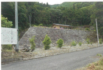
⑱ Ikawa Power Plant Site
