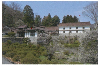
⑤ Nishie Residence Main Building and Other Structures
