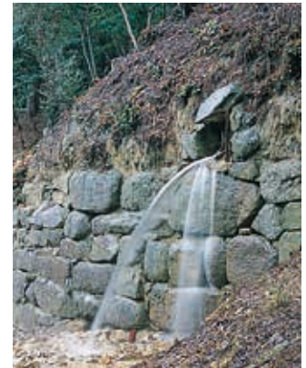
The floodgate in the valley
